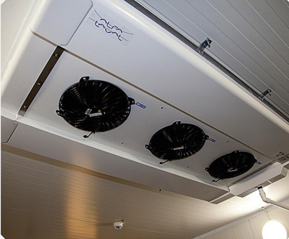
S-Market's cooling system consists of one Optigo CD cooler in the fish cold room (0-2°C or 32-35.6°F), chicken cold room (0-2°C or 32-35.6°F), ready-food cold room (3-5°C or 37.4-41°F), fruit and vegetable cold room (6-8°C or 42.8-46.4°F), as well as three coolers in the terminal area (2-4°C or 35.6-39.2°F).
